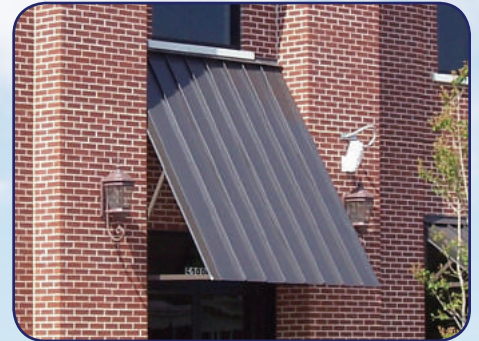
Entrance Awning With Open Ends
