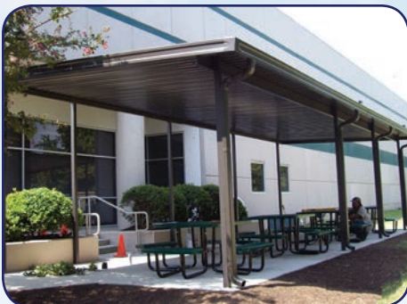
Employee Break Areas
