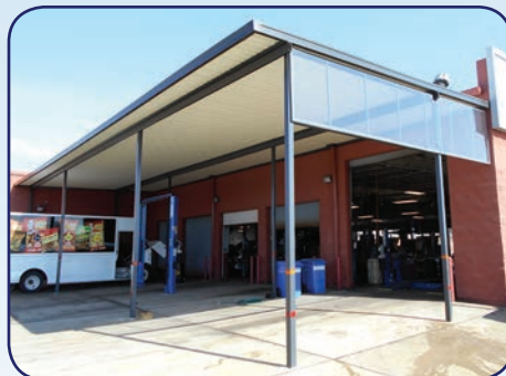
Canopy Using Roll Form Fascia & Decking
