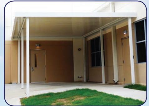
Metal Canopy With Flat Pan Decking
