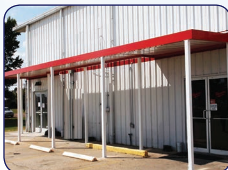
Wall Attached Metal Canopy With Extruded Fascia
