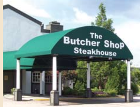
Marquee Entrance Canopy
